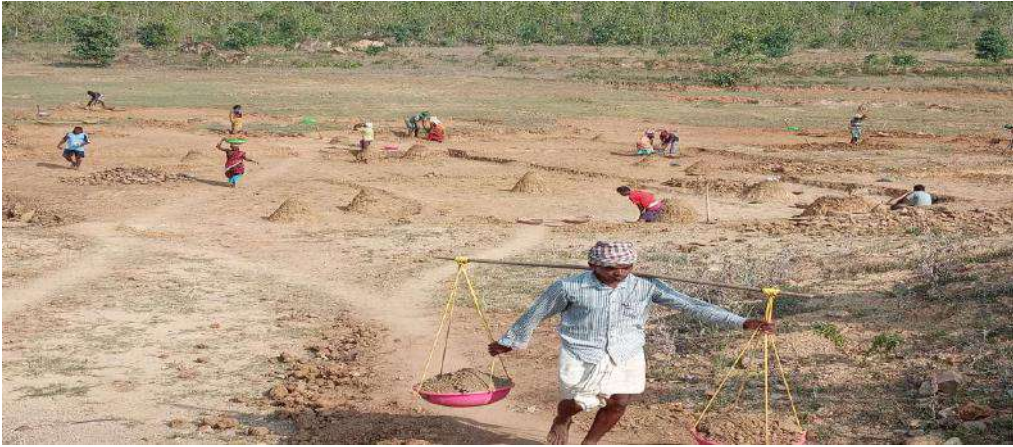
Renovation of Tank in Amsena GP of Nuapada Block
